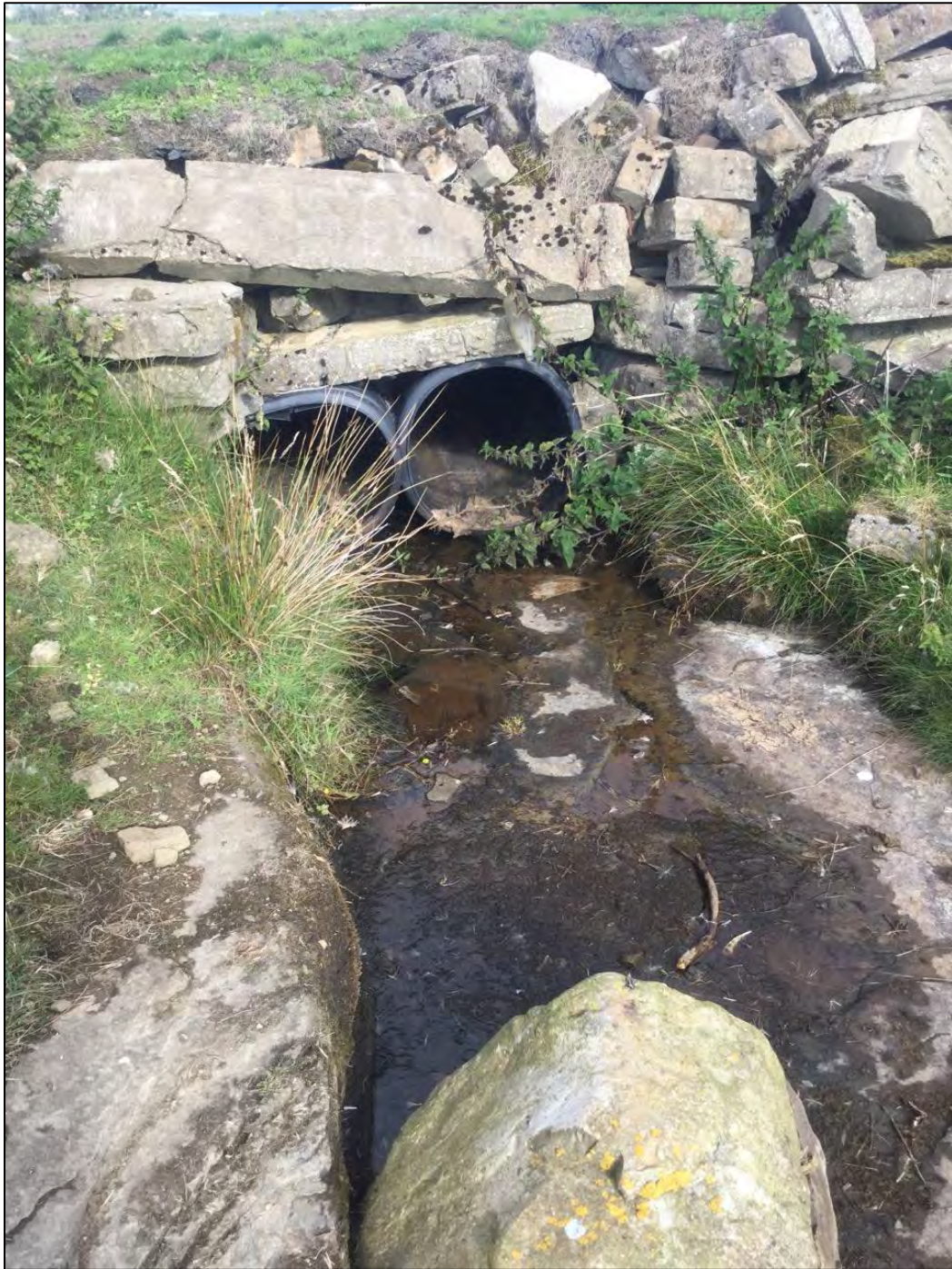
Photo 7. Burn of Brims flowing underneath piped culvert.
