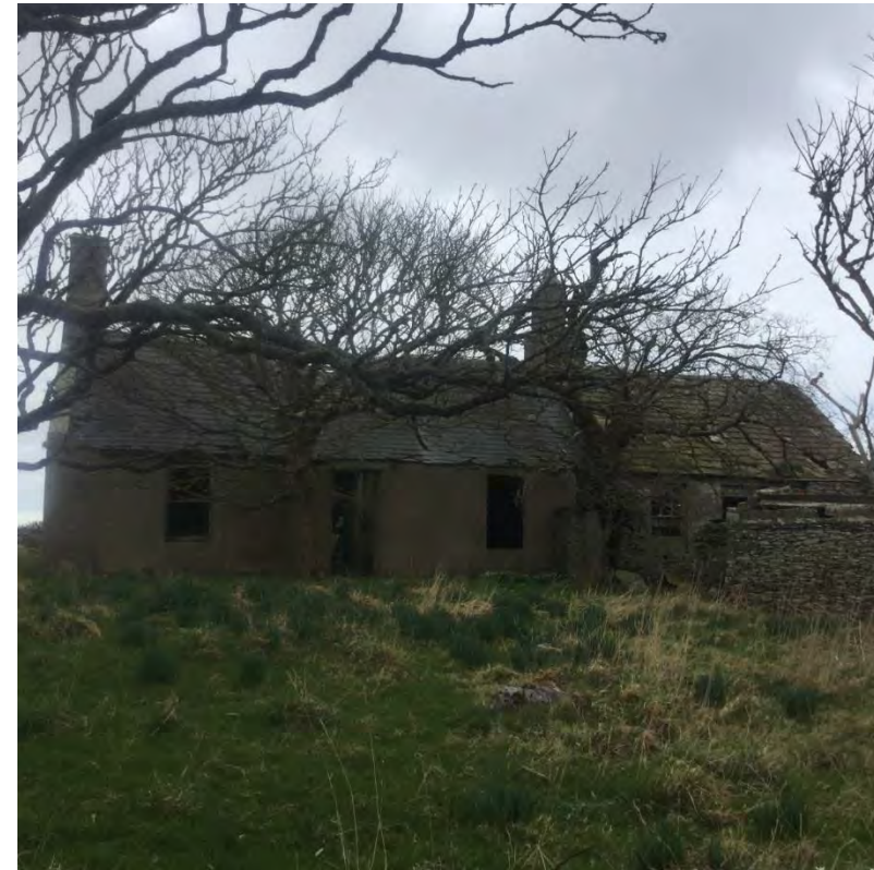
Photo 3 Blackheath Farm house bungalow (north facing)
