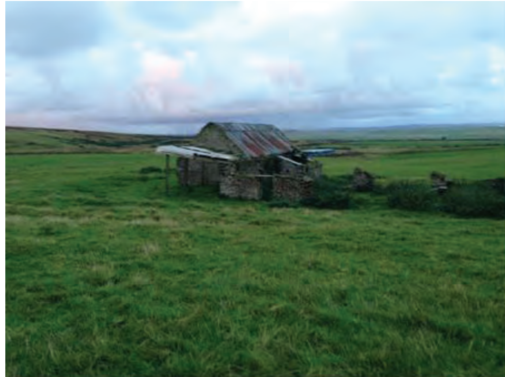
Photo 17. View of derelict building and surrounding improved fields (ND060691) © Stuart Spray
