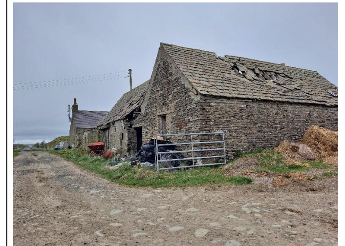
Northern, site facing facade of Hopefield.
