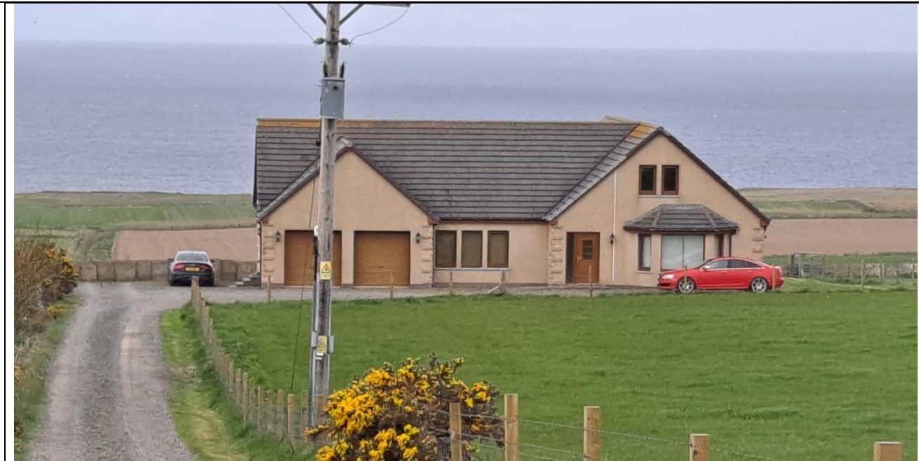
Southern (site facing) façade of Brimmisa House.
