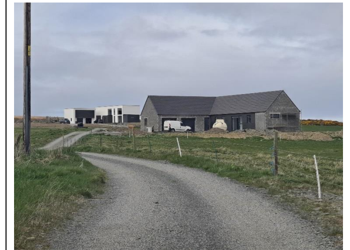
View looking north towards Group 12 (Roan Va in foreground), with site behind.
