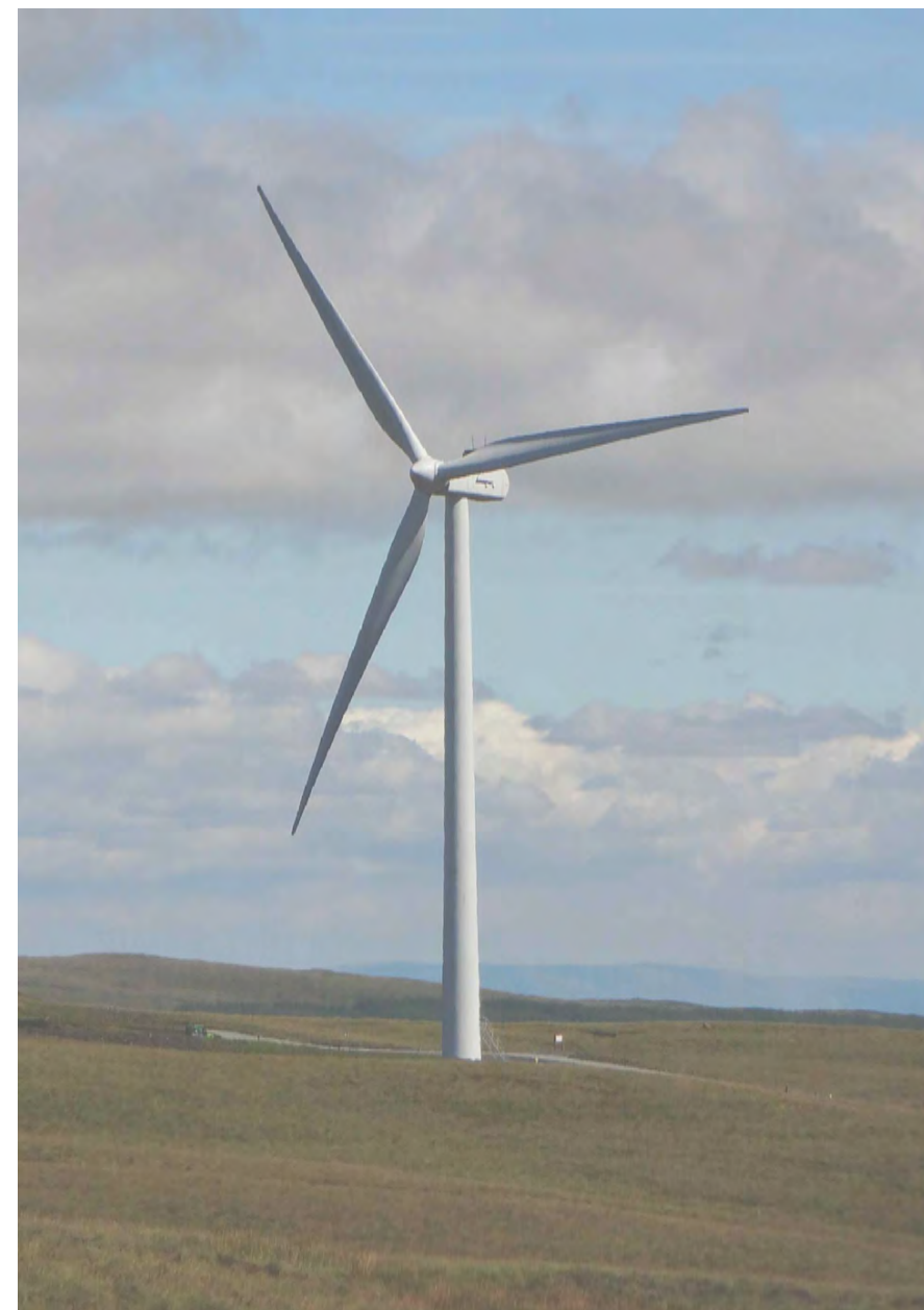
PHOTOGRAPH OF TYPICAL TURBINE
